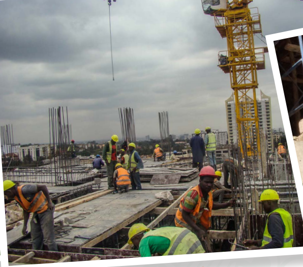
Construction workers laying the foundation
