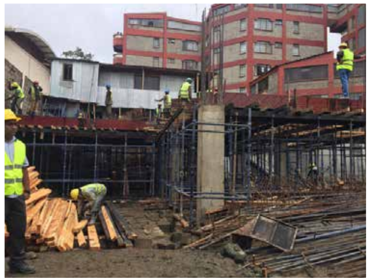
Ongoing construction work at the 850 Chania project site
